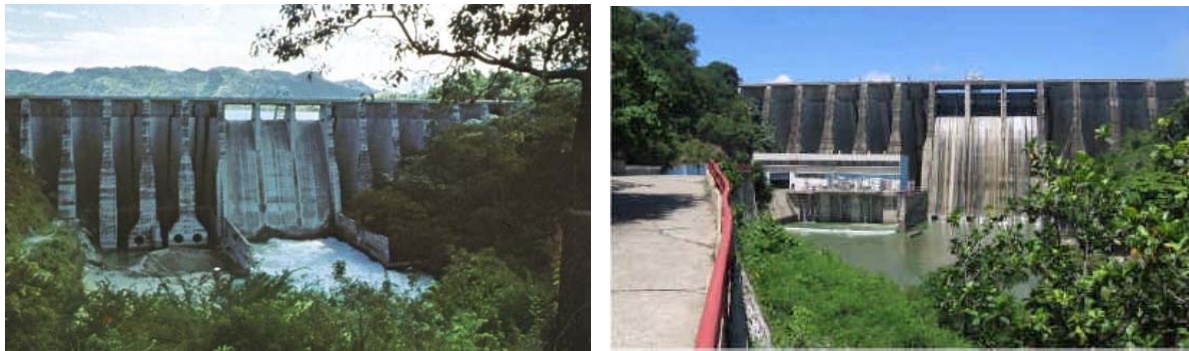
Fig. 1: Péligre dam before powerhouse construction (left) and before rehabilitation in 2012 (right)
