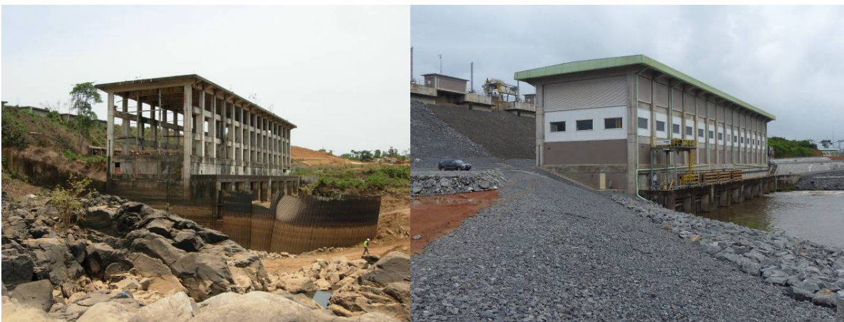
Figure 2 - Power House before (2013) and after rehabilitation (2017)
