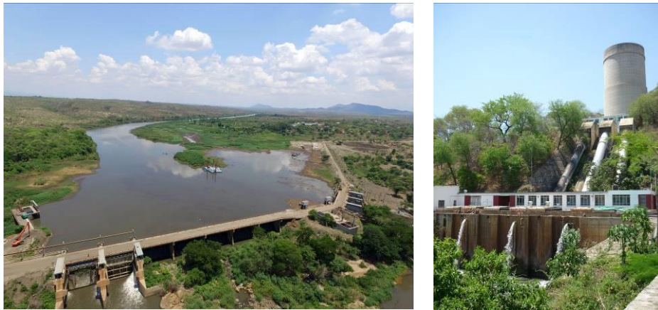
Fig. 1. Left: Nkula reservoir; Right: Nkula A hydropower station before rehabilitation
