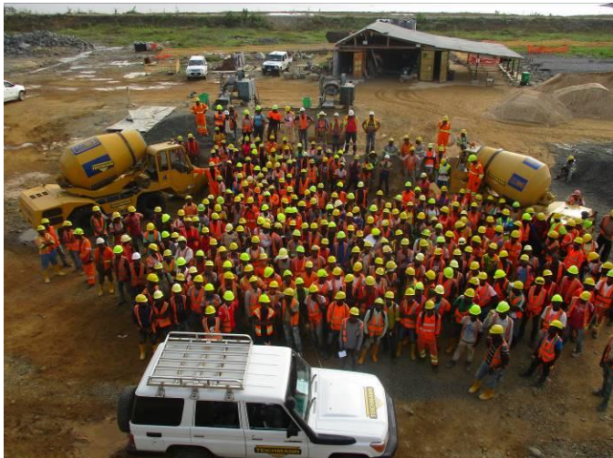
Figure 7 - Local workers employed for the RMC weir construction
