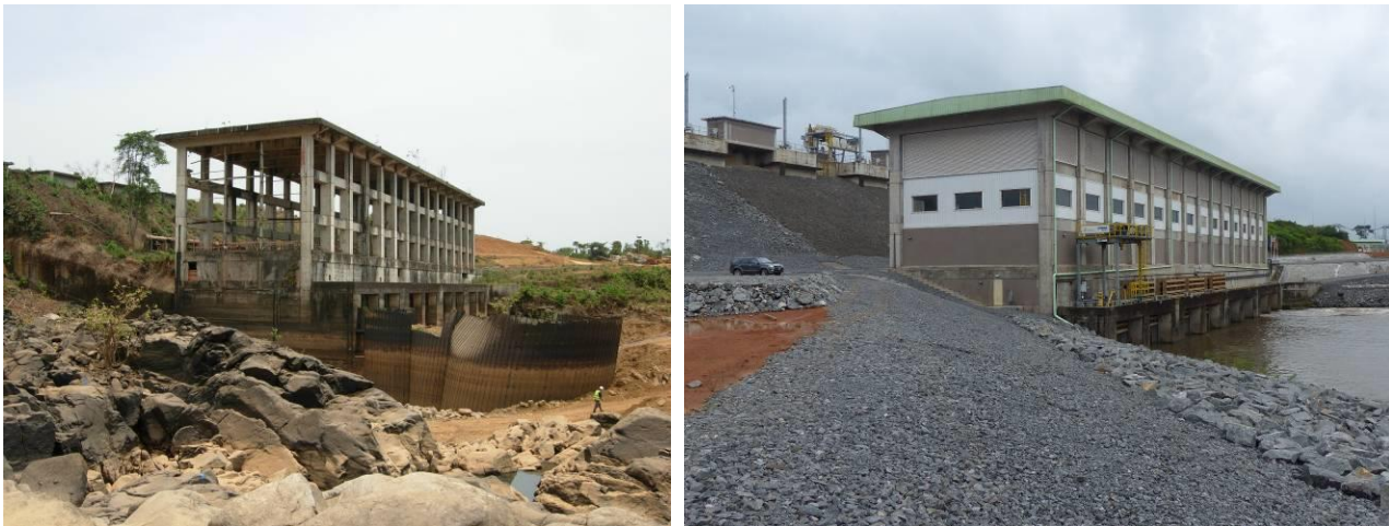
Figure 1 - Power House before (2013) and after rehabilitation (2017)
